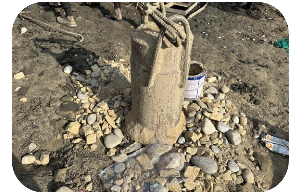
Gravel Compaction
