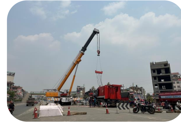
Crane for Lifting
