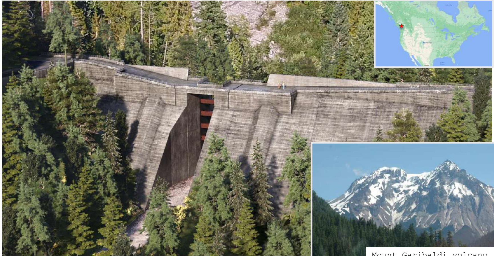
Digital rendering of the Cheekeye barrier. Barrier is about 25 m tall
