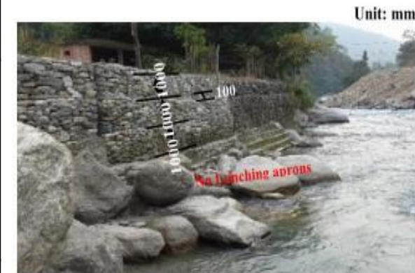
Gabion constructed at Sasaha Khola, Dhading, Nepal
