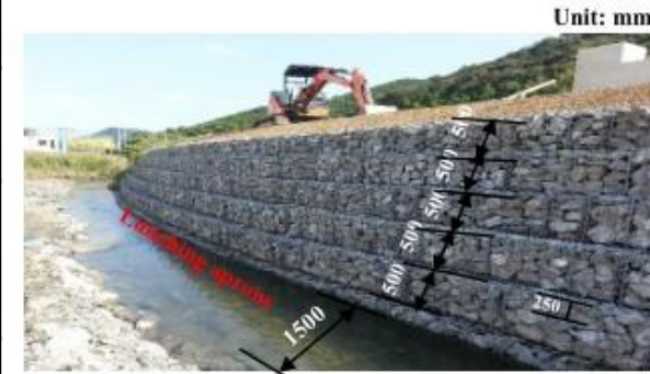
Gabion constructed Minaminotanigawa, Kochi, Japan
