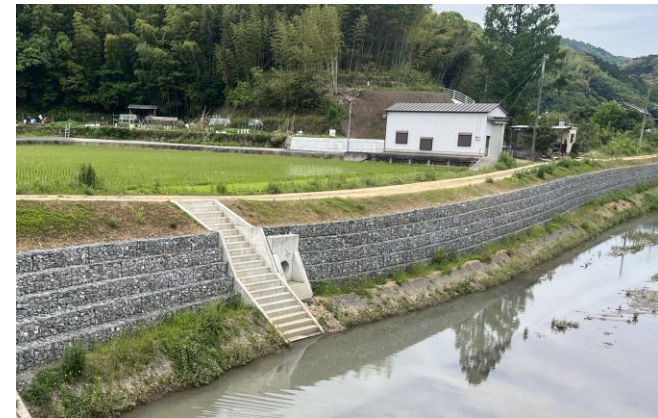
Gabion in Okudakhawa Kochi Japan
