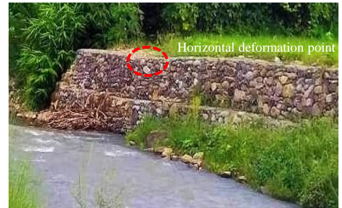
Schematic diagram of gabion based retaining wall deformation
