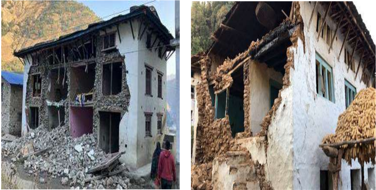
Figure 3: Out of plane failure
