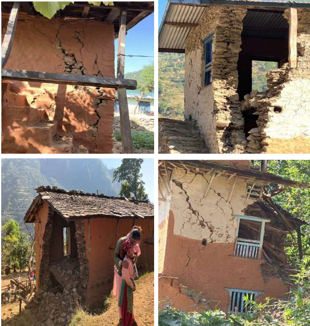
Figure 5: Corner failure
