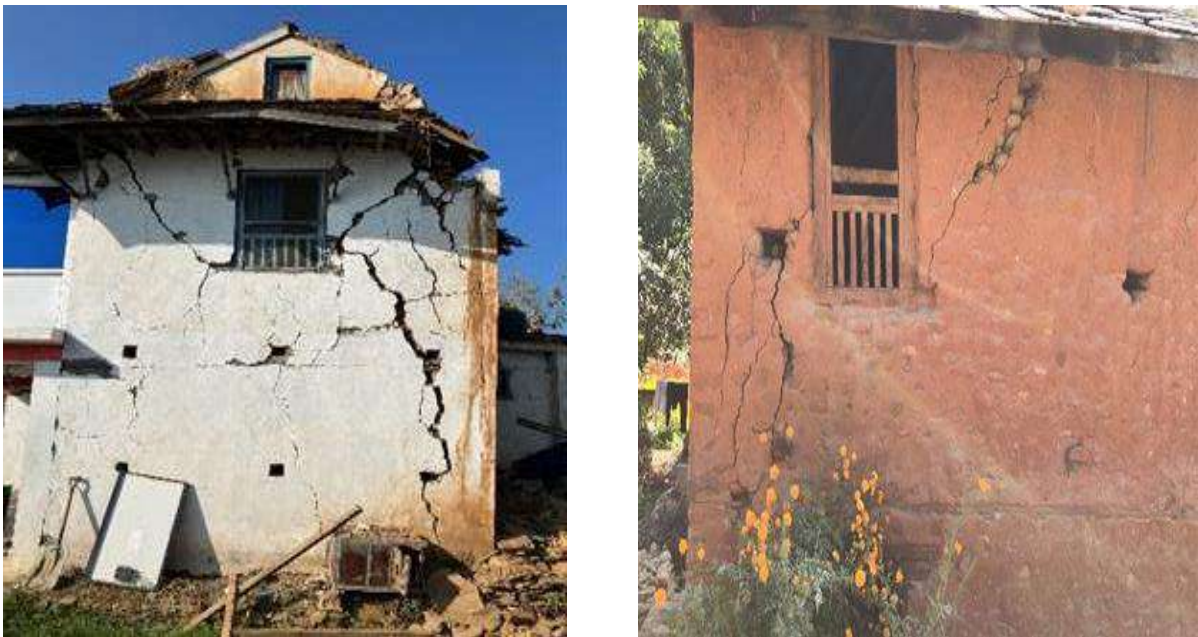
Figure 4: Diagonal cracks
