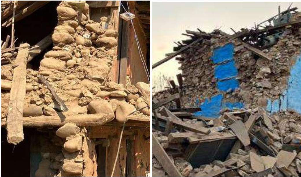
Figure 2: No through stone block in wall thickness
