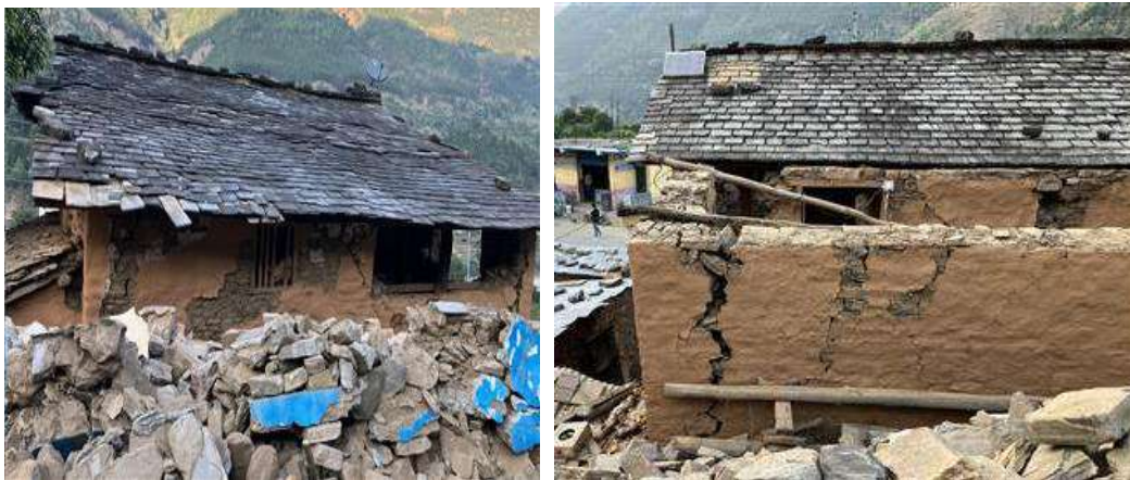
Figure 6: Building with heavy roof weight.
