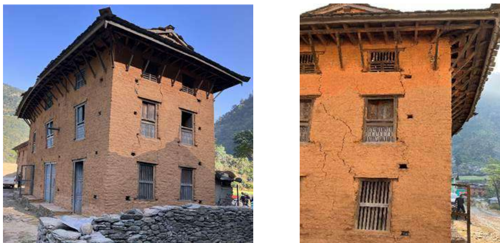
Figure 7: Vertical crack in opening
